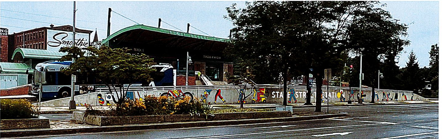
View of the wall from across State Street, approaching from the north
