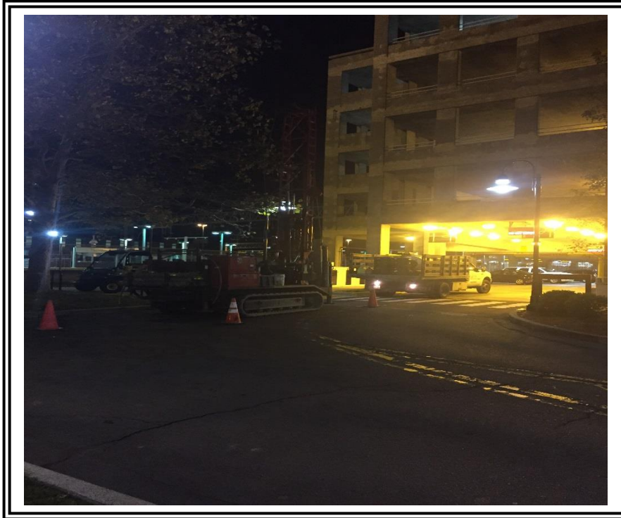
Drilling operations at B-1, looking south
