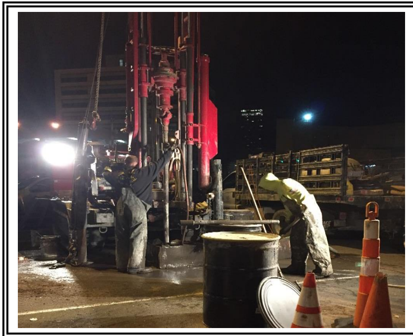
Drilling operations at B-6, looking north
