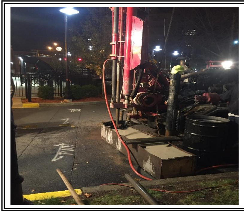
Drilling operations at B-1, looking northwest
