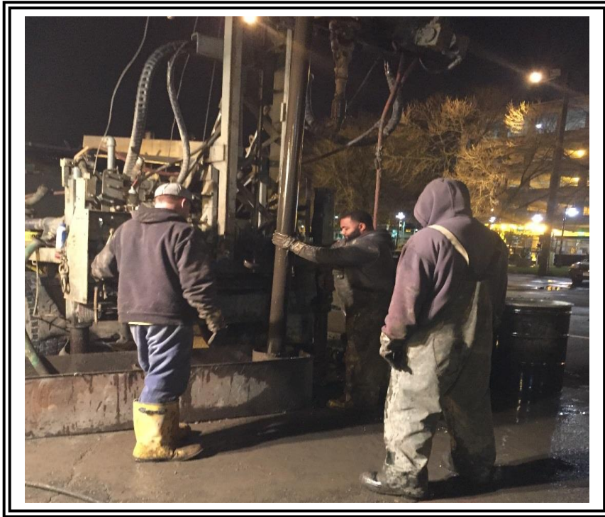
Drilling operations at B-13, looking north
