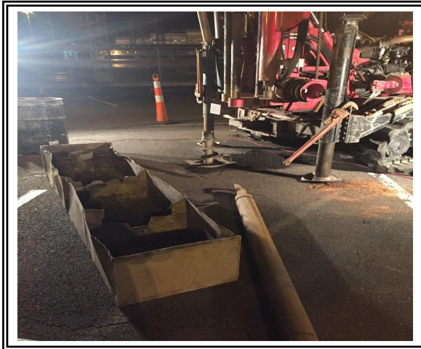
Drilling operations at B-5, looking southeast
