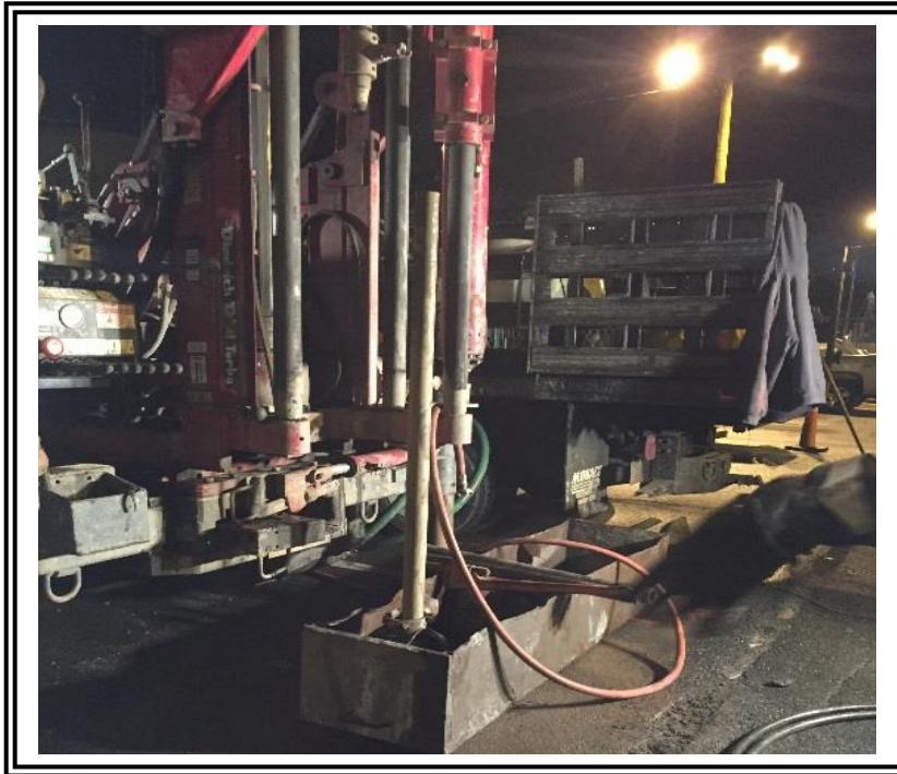
Drilling operations at B-7, looking east
