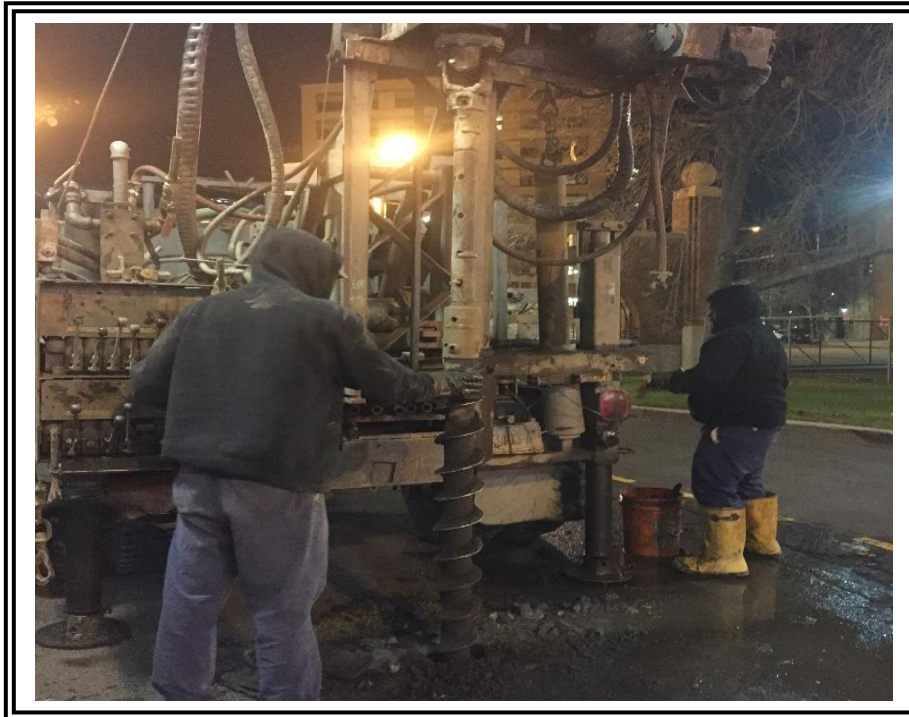
Drilling operations at B-11, looking north
