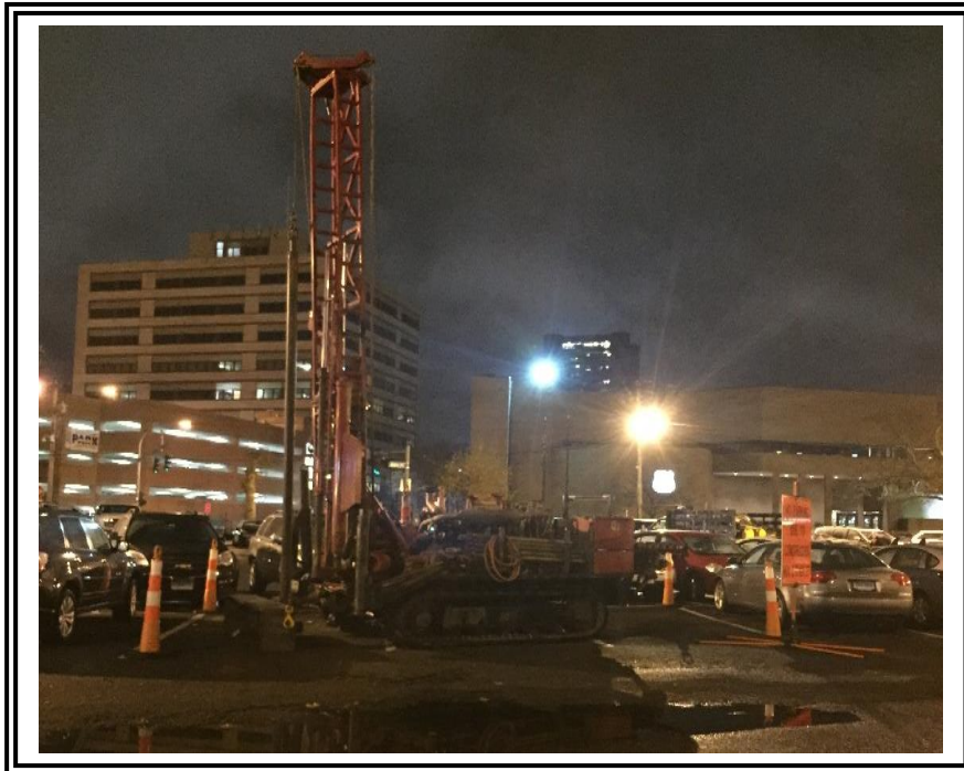
Drilling operations at B-4, looking northwest
